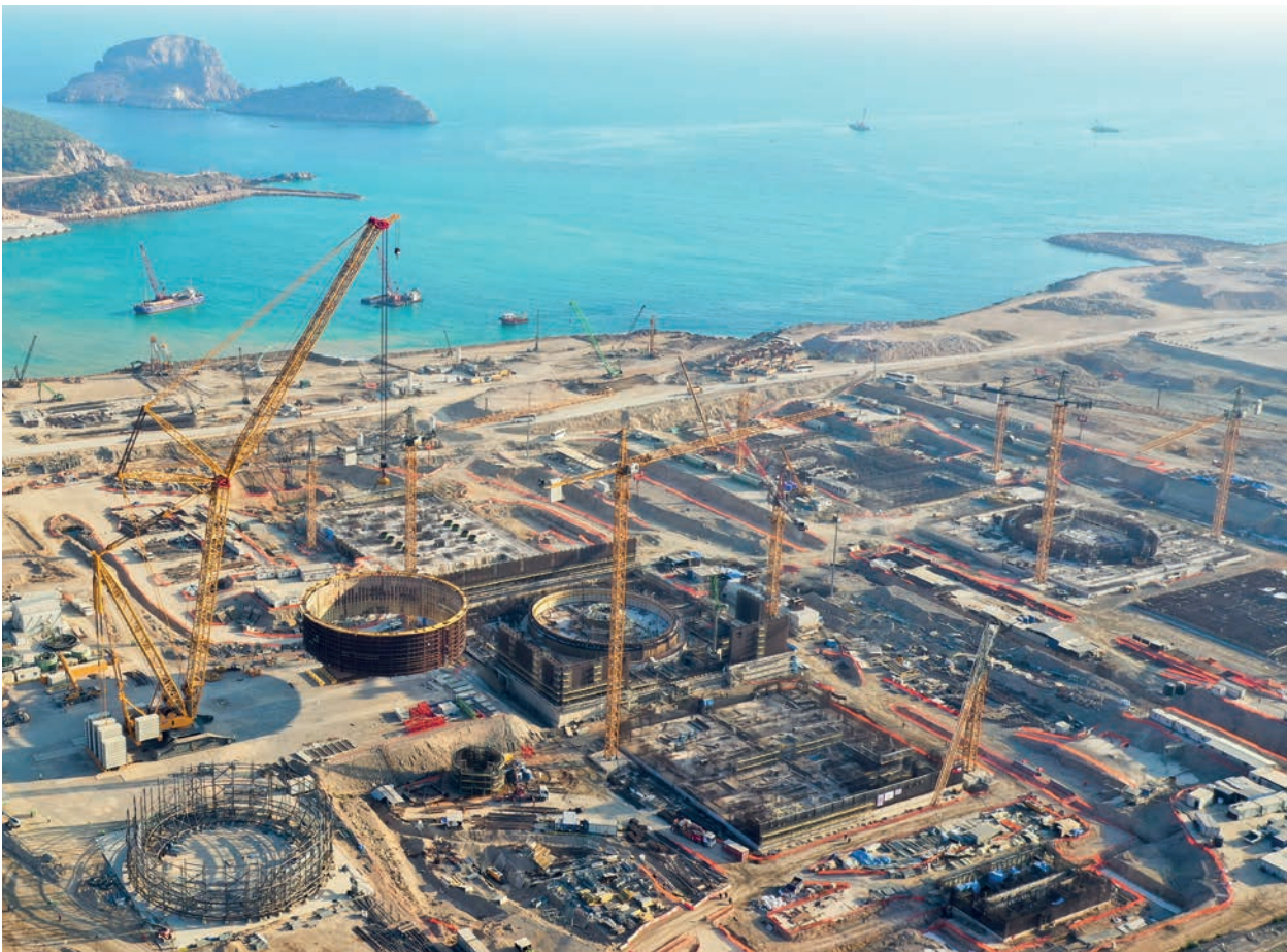
Earlier construction at Akkuyu. (Image: Akkuyu image bank, ROSATOM)
