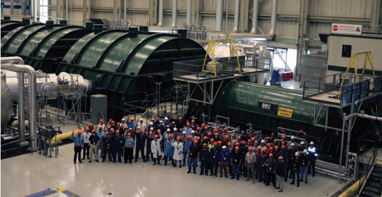
U3 Returned to Service – staff on the Turbine floor photo (Image: OPG)
