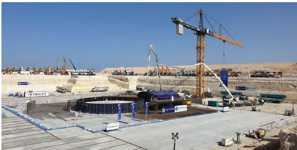
Start of construction of unit 2 at El Dabaa (Image: Rosatom)
