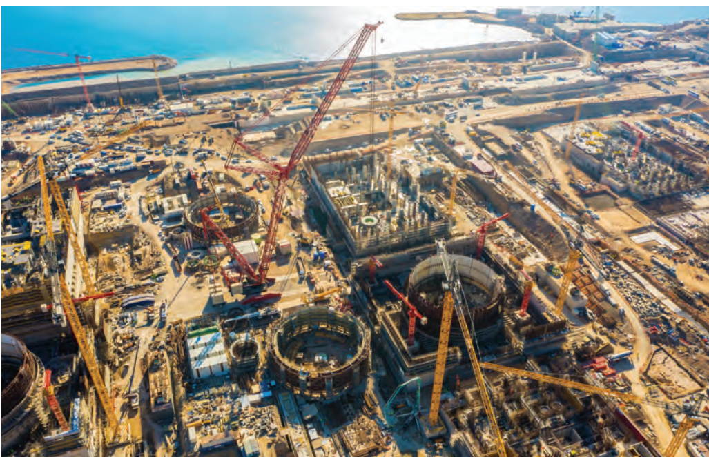
Unit 3 under construction (Image: Akkuyu NPP)
