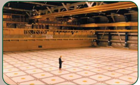
ILW interim surface store
